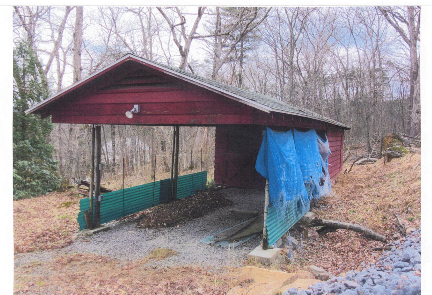
PICTURE OF GARAGE (EAST SIDE)
