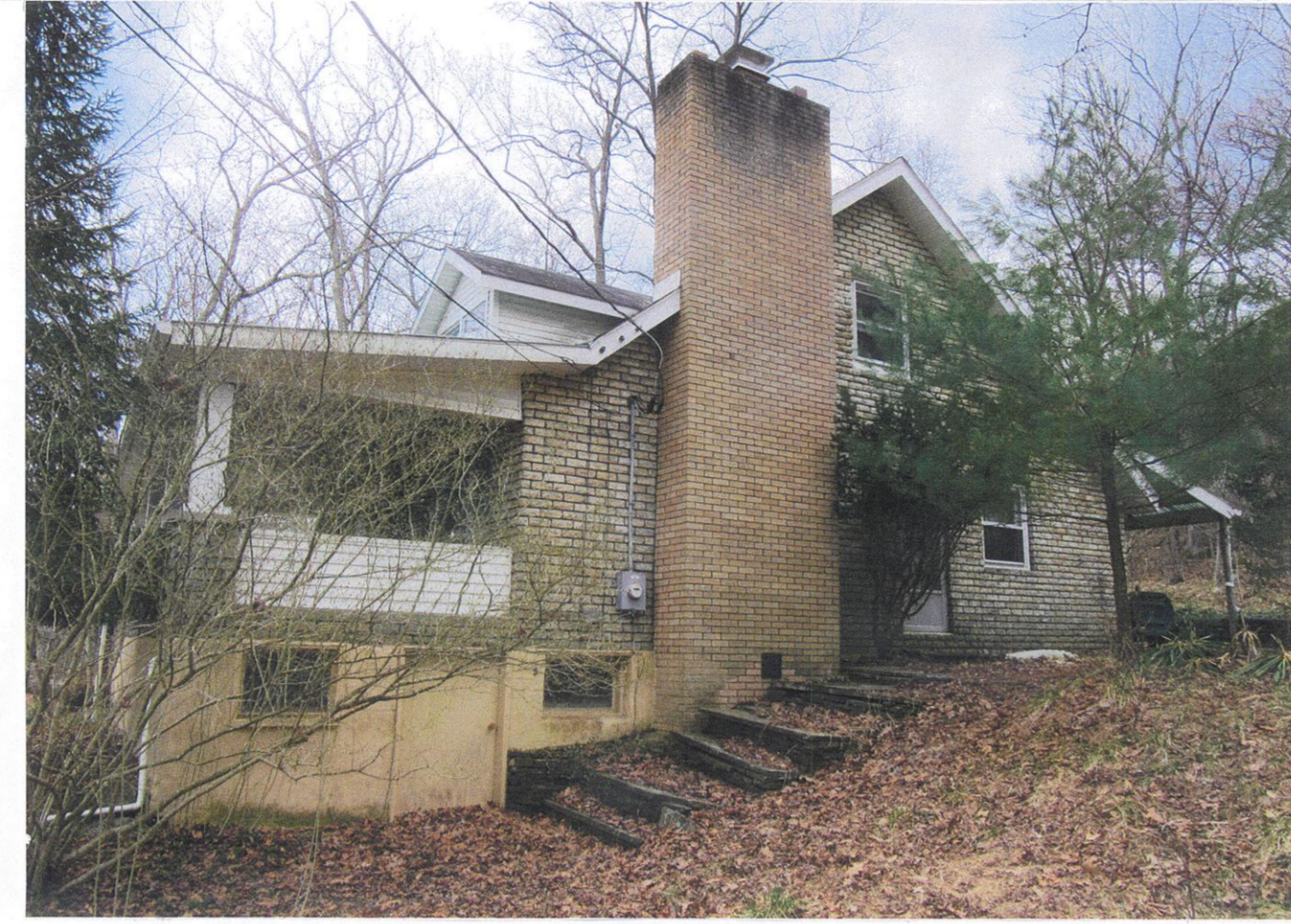
PICTURE OF HOUSE (EAST SIDE)
